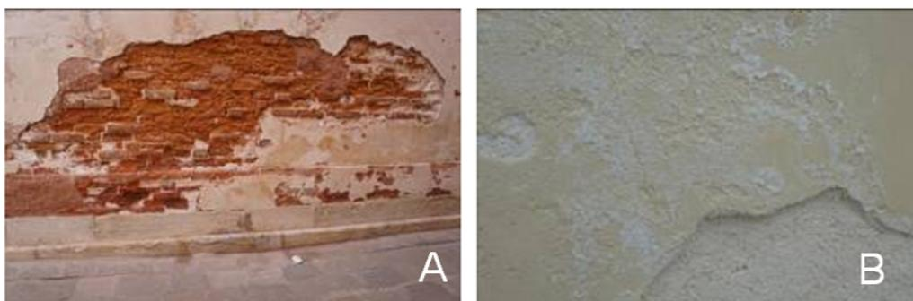
Fig.4 Examples of degradation due to the action of rising damp and salt solutions; A) detachment of the mortar due to the crystallization of salts , B) presence of salt efflorescences over the render.
